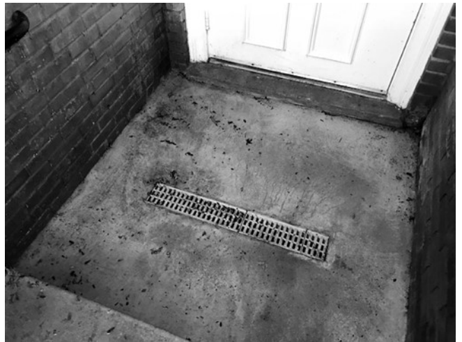
New grates with large holes were installed to facilitate drainage.
