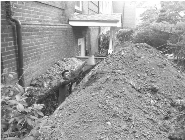
Workers dig a trench to replace the drainpipes and install cleanouts.
